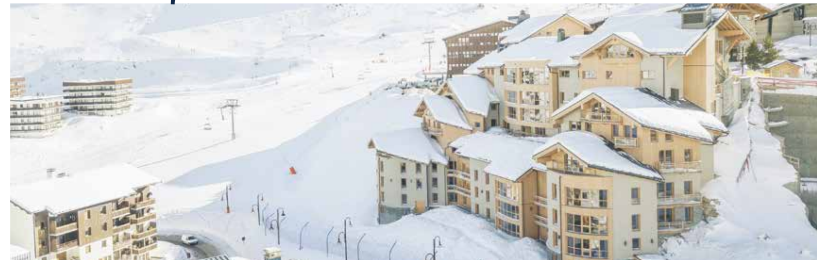
The Group contributed to building the four-star Le Taos Hotel in Tignes
