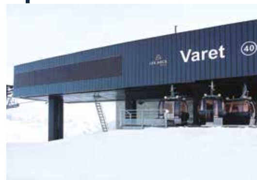
At an altitude of 2,679 metres, the Varet station in Les Arcs has been equipped with solar panels
