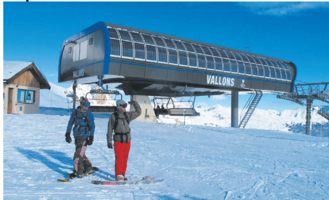
Solstatiar on panels on the Vallons chairlift
