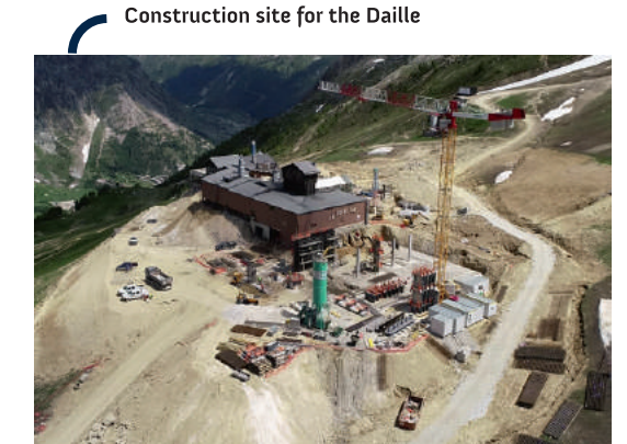
Construction site for the Daille
